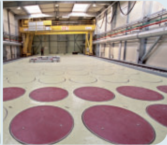
Wells for the storage of medium-level radioactive waste
