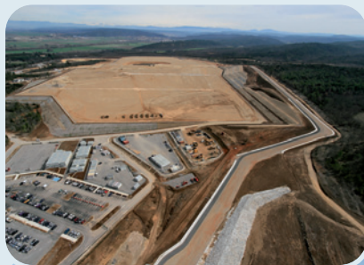
The 40-hectare platform was developed to accommodate the facility
