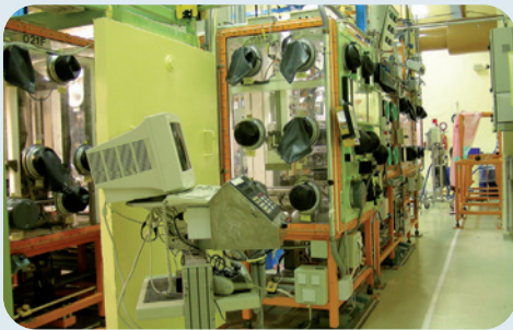
The Plutonium technology facility undergoing dismantling operations
