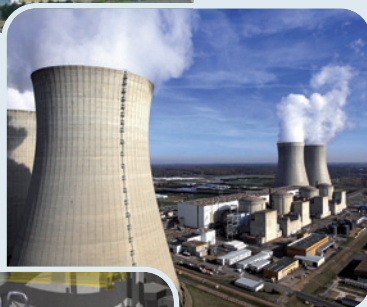
Dampierre-en-Burly: Generation 2 plant
