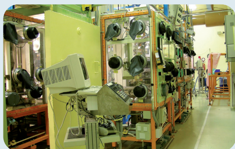
The Plutonium technology facility undergoing dismantling operations
