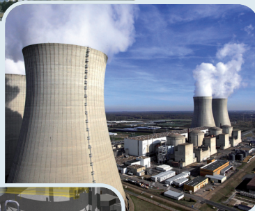
Dampierre-en-Burly: Generation 2 plant
