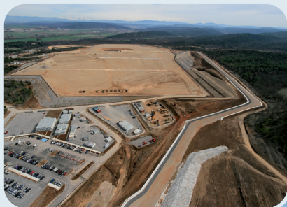
The 40-hectare platform was developed to accommodate the facility
