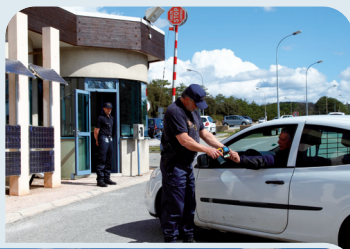
Guarded access to the site
